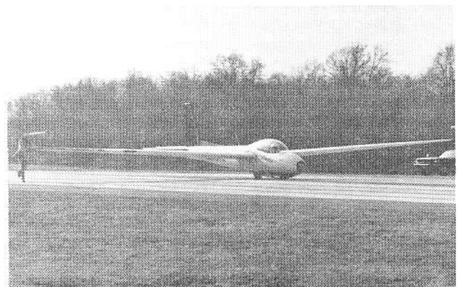
Figure 2: Instrumented Schweizer 2-32 Sailplane
