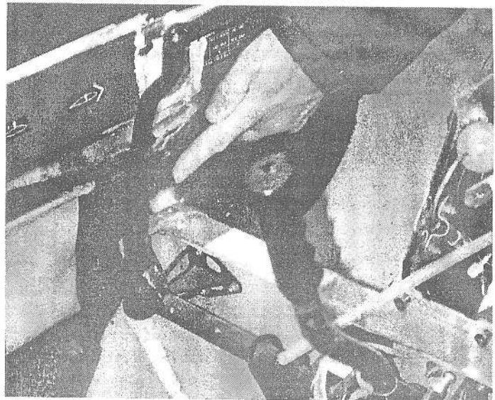
Failure in tension of transverse bulkhead attachment to the cockpit side wall.
